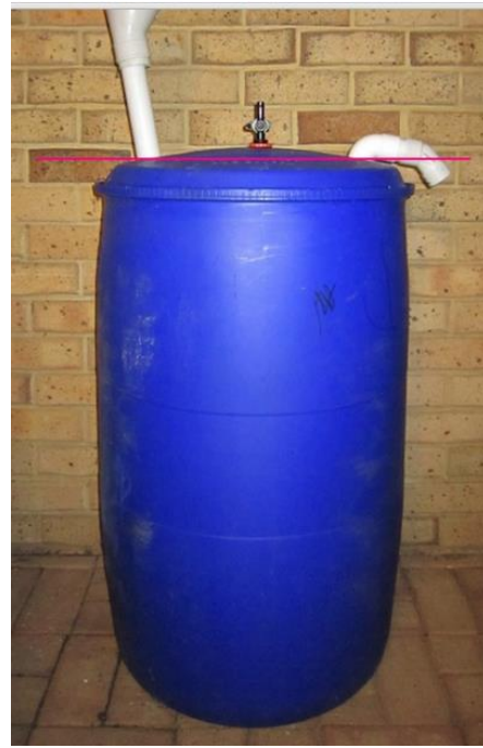
Figure 6b: the water level of the collector should be below the marked line
