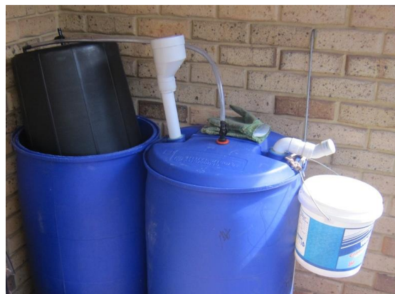
Figure 8: The completed homemade bio gas unit
